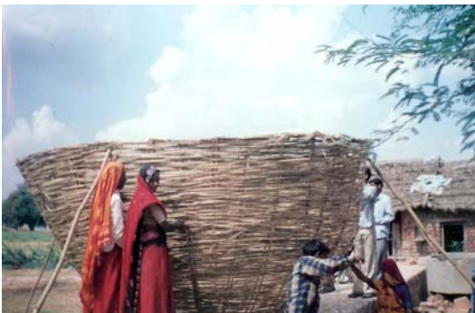
Some of the important stages of practical training on fabrication (splitting, strips making and weaving etc) of bamboo structures to poor landless women with in their own (Nagla Banjara) village, to be used for building Grameen Bandhu Plant (GBP)
