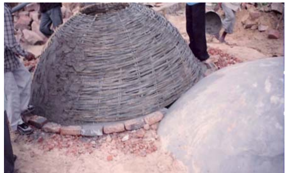
Some of the important stages of practical training on fabrication (splitting, strips making and weaving etc) of bamboo structures to poor landless women with in their own (Nagla Banjara) village, to be used for building Grameen Bandhu Plant (GBP)
