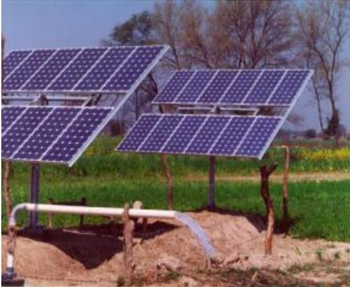
A solar photovoltaic water pumping system consists of a photovoltaic array mounted on a stand, and one of the following motor-pump sets compatible with the photovoltaic array. The photovoltaic array converts the solar energy into electricity, which is used for running the motor pump set. The pumping system draws water from the open well, bore well, stream, pond, canal etc.
